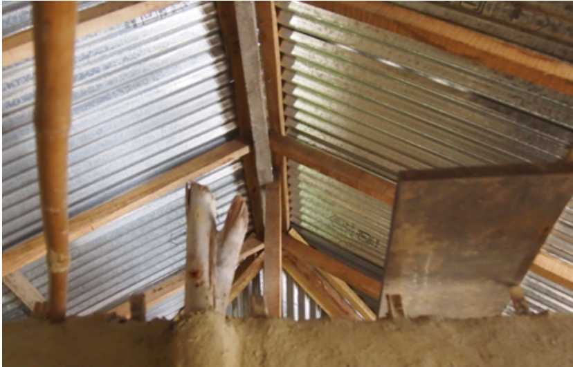
The local shelters were tin-roofed, offered virtually no insulation against heat, cold, and outside noise.
