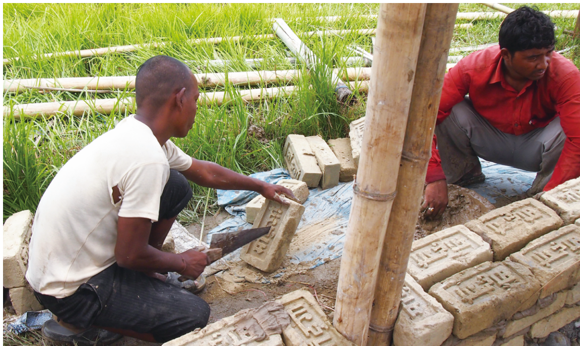
Construction of a house made from mud bricks—one of our three prototype homes. To close the gaps between the mud bricks and the bamboo pillars, we filled them in with thin pieces of bamboo strips and kept them in place using wire.
